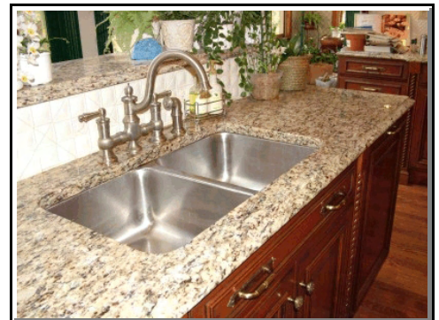
A granite top like this must be installed on kitchen cabinets that are level and sturdy. PHOTO CREDIT: Tim Carter
