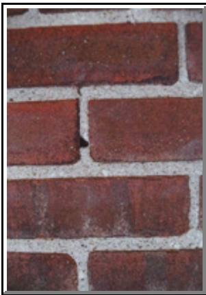
The color of the grains of sand makes a huge difference in mortar color once the actual cement paste wears away.
