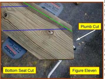
just at 11.5 inches. Furthermore, if you could put a tape measure on this same pencil line, it would be 7.5 inches long from where it touches the framing square to where the tip of the white arrow is. Once again, **your riser height may be different**!
