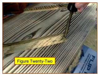
ers. This is actually the underside of the stairs once the treads are installed in the stringers. You could create rectangular mortises that perfectly matched the shape of each tread, but that is one heck of a lot of work. If you feel you have the time and inclination, go for it.
