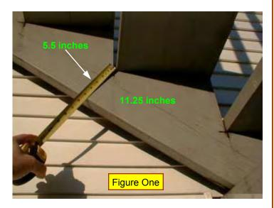
Take a look at Figure One. It is a set of steps located not too far from my home. It is built as I see many stairs built. The carpenter laid out the risers (the vertical dis-
