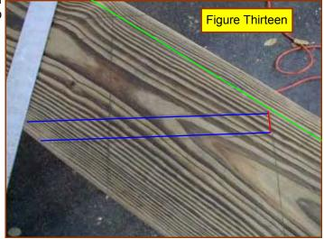
ing to be cut out to a depth of just one-half inch. It will make a perfect recessed area for each tread to fit into.
