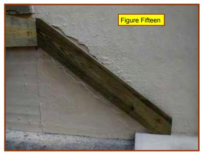
colored lines. If I had left this triangle of wood on the stringer, it would project up above the surface of the landing, deck or second floor or whatever the finished flooring is. Remember, the length of the **red** line in Figure Fourteen is 7.5 inches or the height of my risers. Your riser height may be different.
