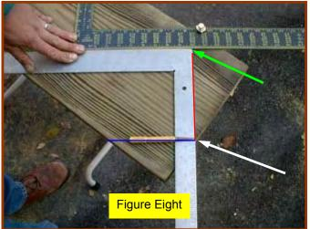
1.5 inches. A similar 1.5 inch border needs to be added to the front of the first riser. You can see a similar border added in Figure Nine. The distance of the border in Figure Nine is more
