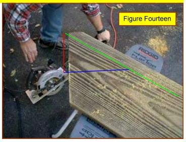
I also made a secondary cut at the top of the stringer. The 1.5 inch setback indicated by the green line is the cause behind this cut. In Figure Fourteen, can you see how the top of the stringer is parallel with the blue line? The blue line represents the top of the last tread. Before I cut the top of the stringer, it came to a point. I have outlined the missing piece with magenta
