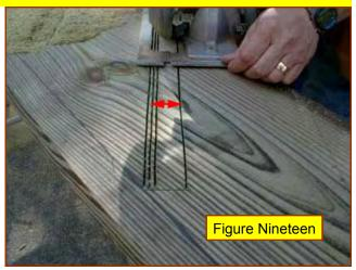
make the outer cuts. If the mortise is too narrow, it will be impossible to fit the tread into the mortise. If you are sloppy and cut it too big, it will look very bad once the stairs are assembled. It is easy to get it right, just check and double check measurements before you make your cuts.
