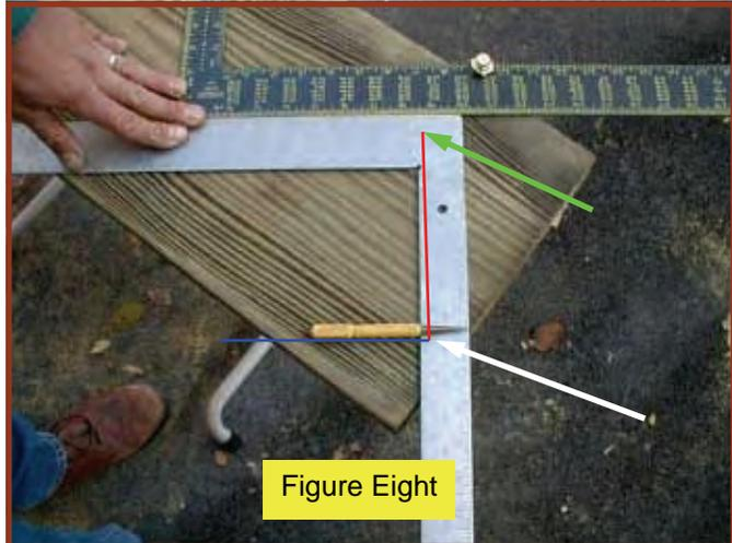
than the border distance from the tips of the treads to the top edge of the stringer. I cut it this way for this set of stairs so that the vertical face would not be too terribly high. On outdoor stairs, I prefer to have the distance between the tips of the two green arrows the **same as the distance between the tips of the treads to the top edge of the stringer**. In the stairs we are building now, I will make this distance 1.5 inches.
