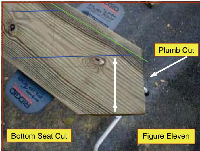
Figure Eleven shows you the bottom of the stringer once I have cut along the pencil lines. This photo is actually a little out of order as it shows the layout lines of the treads already complete. I am just about to show you how to do that. But I wanted you to see how the cuts make sense.
